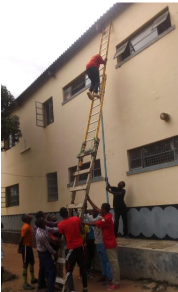
Figure 1: Climbing a two floor Building to Install a Receiving antenna
